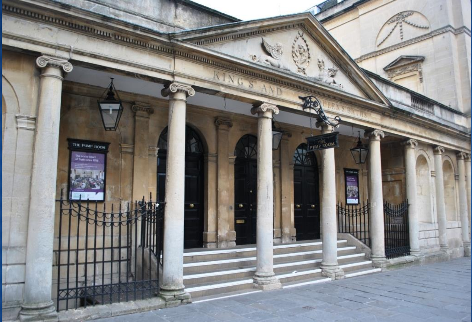
South Colonnade, Pump Room
